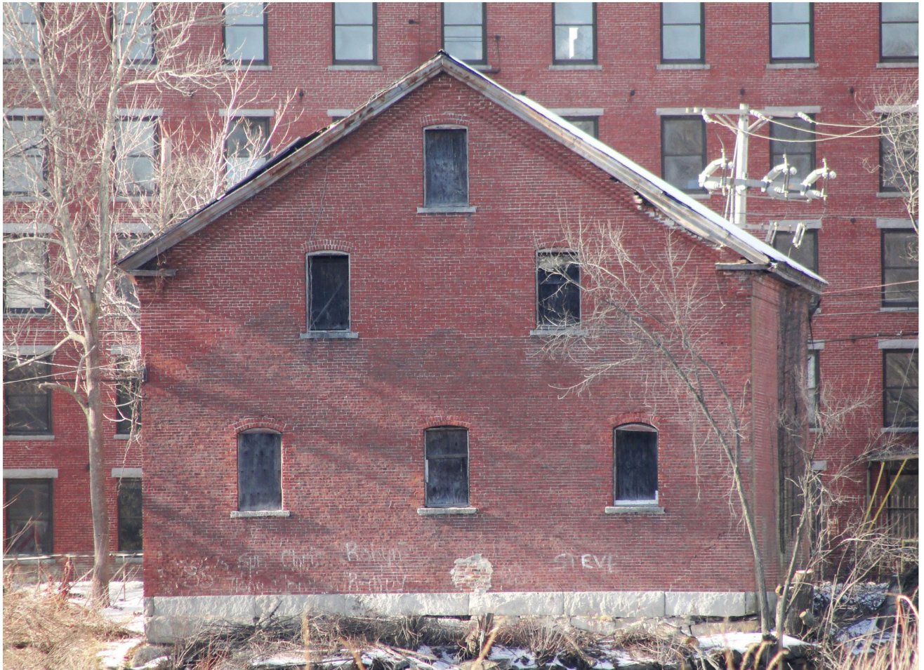
Storehouse No, 2, 2 Old Elm St, Billerica - east elevation, Jan 2016.
