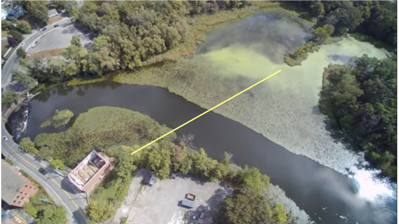
Location of 400' long floating towpath on summit pond between 2 Old Elm St and causeway. Dilapidated roof has been removed from 2 Old Elm.
