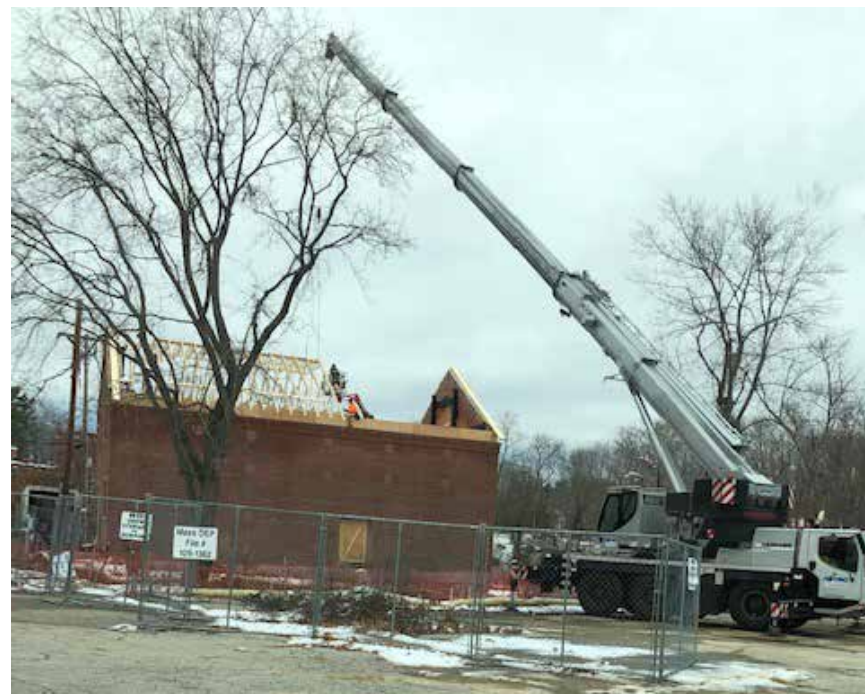
The ever-present costly crane hoisting the roof trusses into place
