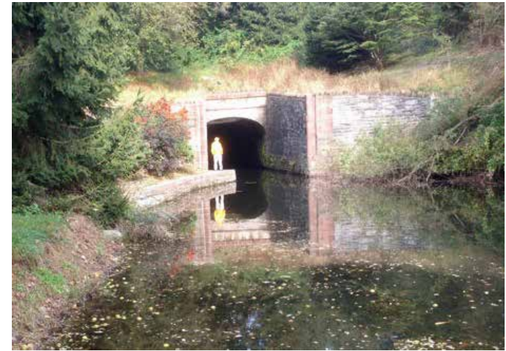
Figure 2. Union Canal tunnel, Eastern Portal
