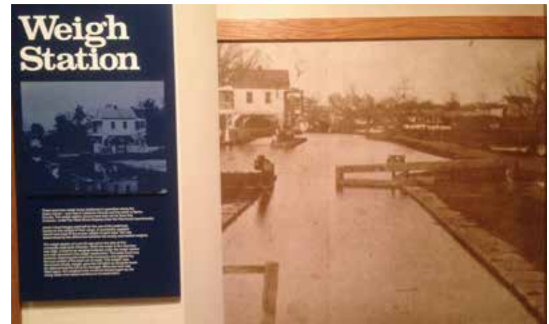
Figure 9. Union Canal Weigh-Lock
