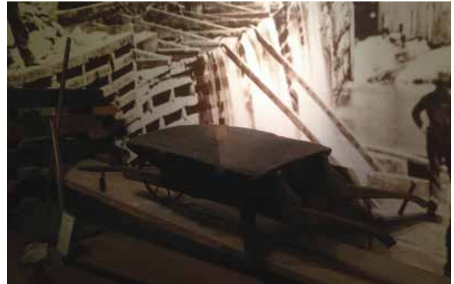
Figure 10. Timber Crib Dam and wheelbarrow
