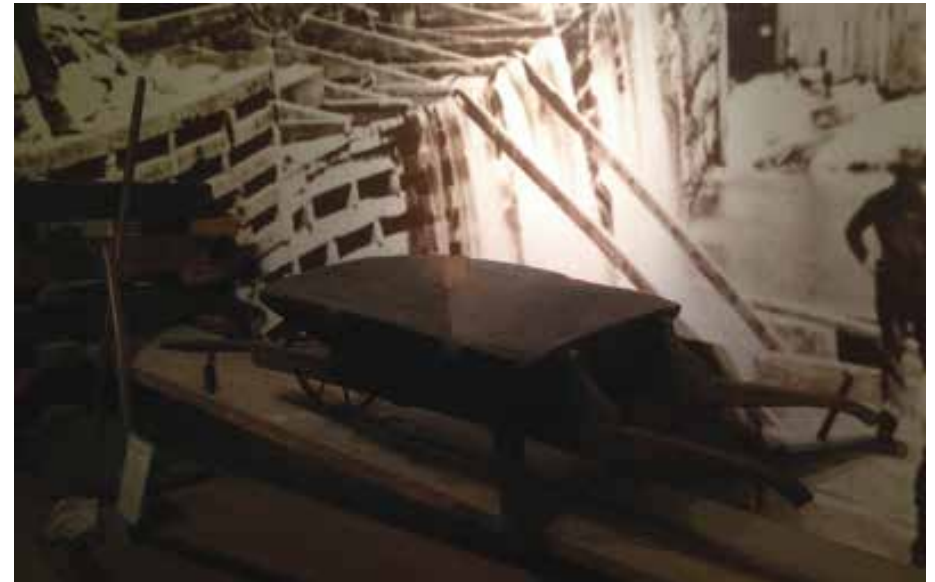
Figure 10. Timber Crib Dam and wheelbarrow
